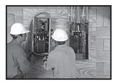
Protect against impact and mount the switch vertically to a rigid support structure. Make sure the switch is level and plumb.
